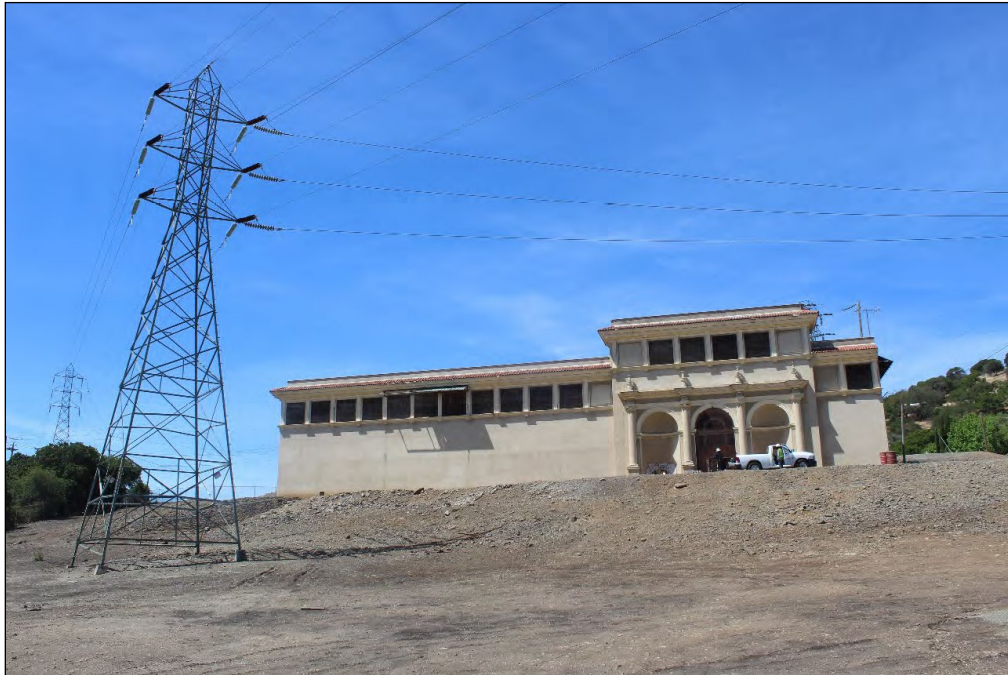
Photograph 1: The Cordelia Substation, camera facing west. April 29, 2021.
